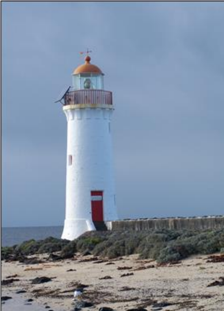
Port Fairy Lighthouse, Great Ocean Road, Victoria
